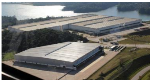
Global Logistic Properties owns this distribution hub south of São Paulo.
